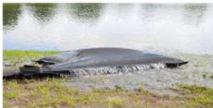
Figure 5-1 Silt Trap Measure at Existing Wheel Wash
